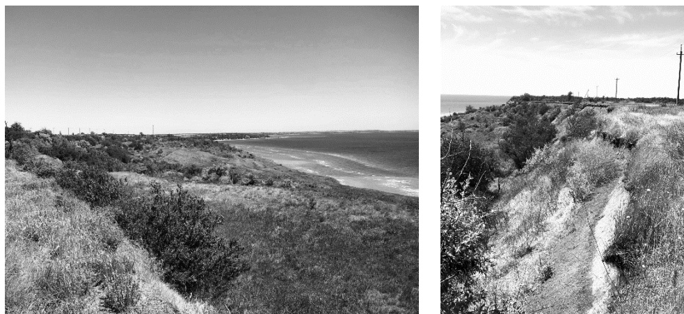
Fig. 7. Landslide coast near Zmeiny Cape (site 22), Belosarayskaya Bay
