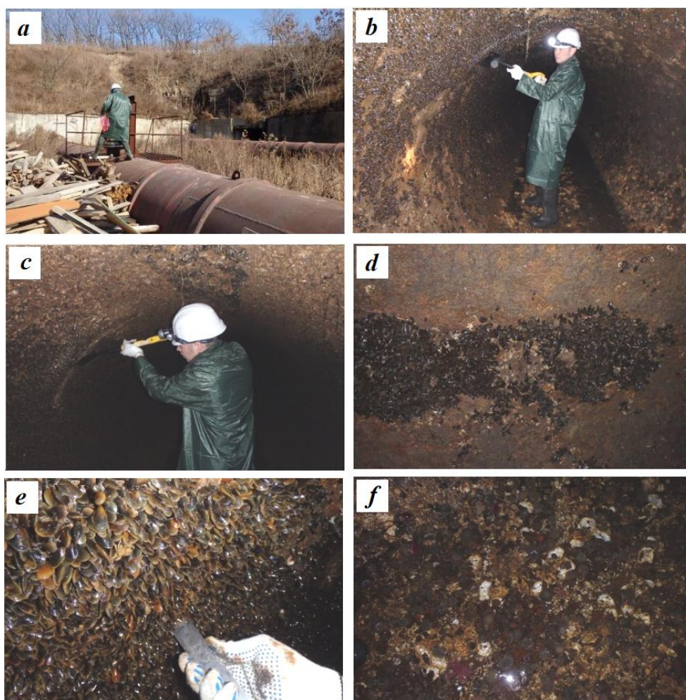
Fig. 2. The sampling process and general view of fouling of the water intake tunnel of CHP-2 in its different sections: a – beginning of the tunnel inspection, b – fouling by sessile polychaete worms of the genus Hydroides , c – test cleaning of the wall to assess the fouling intensity, d – mussel fouling, e – continuous mussel fouling of the tunnel, f – oyster fouling on the tunnel bottom
