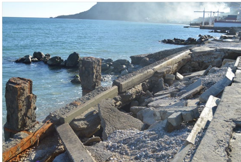
Fig. 8. Reserve filling area. Photo 2021
