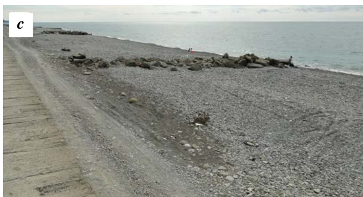
Fig. 4. Use of natural stone in Russian hydrotechnical construction: a – rubble-mound revetment at the right bank of the Nechespsukho River in the village of Novomikhailovsky (the Krasnodar Region); b – a rubble-mound groin with traverses in the village of Nebug (the Krasnodar Region); c – partly ruined rubble-mound groins at the Tuapse – Sochi section
