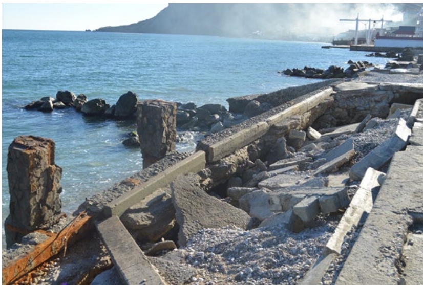
Fig. 8. Reserve filling area. Photo 2021
