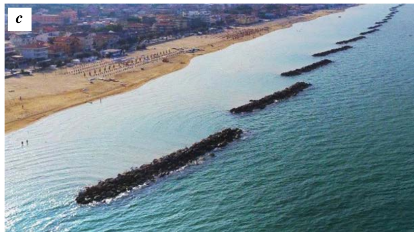
Fig. 2. Examples of coastal protection using natural stone: a – stone sloping revetments, Oregon (the USA); b – stone sloping revetments, Cyprus; c – breakwaters on the Italian Adriatic coast
